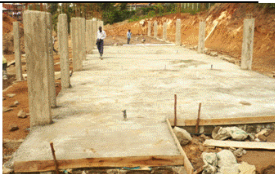
Building progress of the of the new primary school
