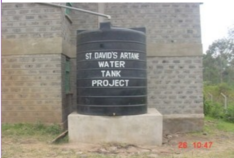
A complete 10000 litres rain water harvest tank initiated by an Immersion group from St. David's Artane in BBCEC in 2010
